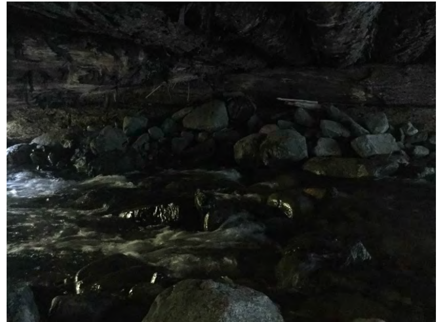
Right Bank Abutment
