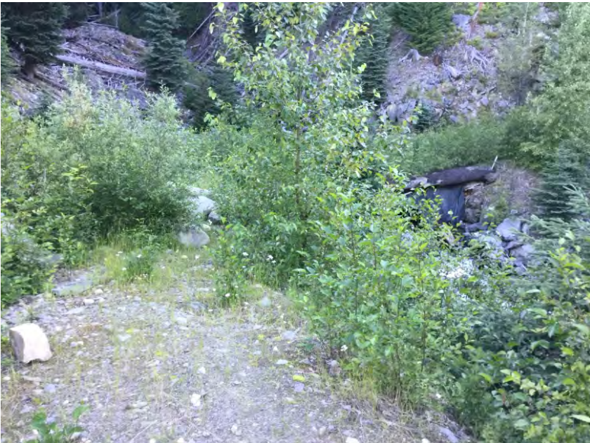
Right Approach Facing Bridge
