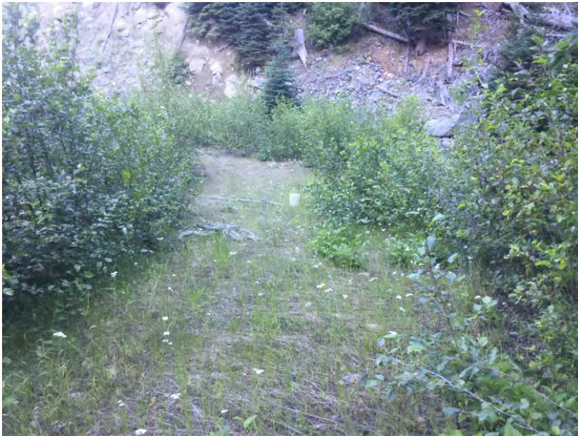
Left Approach Facing Bridge
