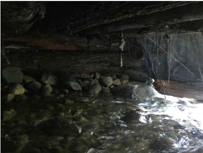
Left Bank Abutment
